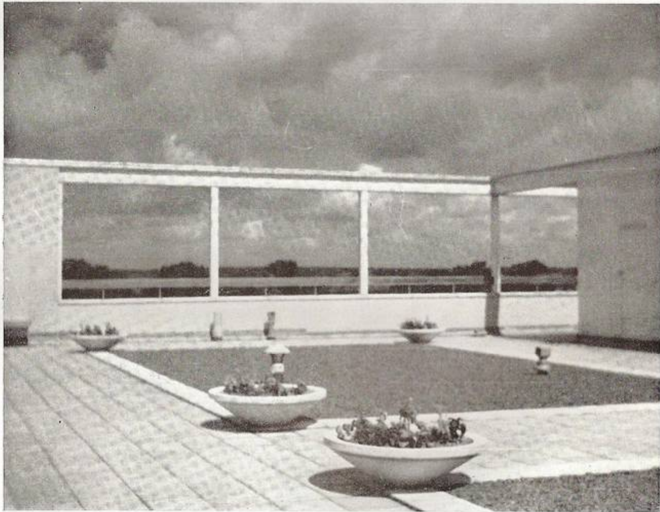
ROOF GARDEN, SCIENCE SCHOOL
